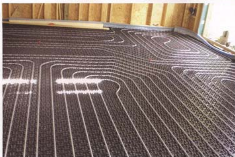
Above: Apart from the render, the exterior of the house is complete, although the landscaping has far too go. Left: Aron laid the complicated network of underfloor heating cables himself
